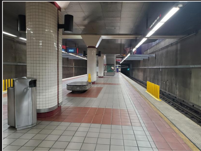
Overnight pressure washing, detailing, and LED lighting upgrade
