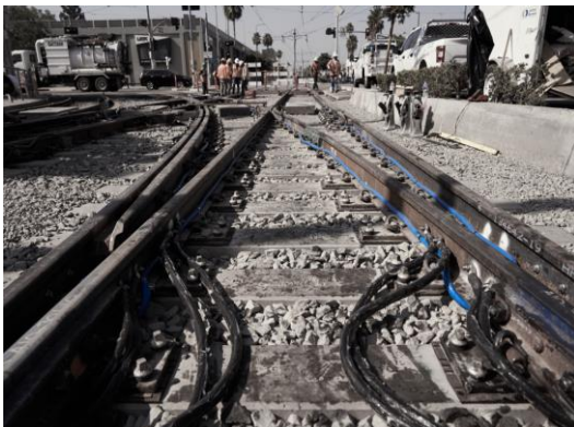
Expo Junction Trackwork
