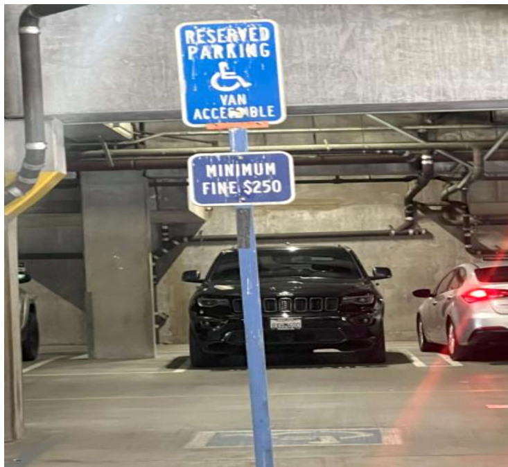
Picture 14 3/11/2026 - Union Station Worn Out Sign/Some Deterioration
