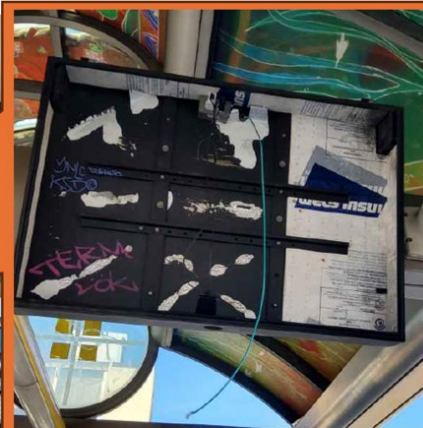
BEFORE: Persistent offenders would stand on the original bench partitions to steal real-time digital displays and cables, then re-wire extension cords to the hiding area behind for unauthorized use, resulting in loss of customer information and $10,000+ in damage.
