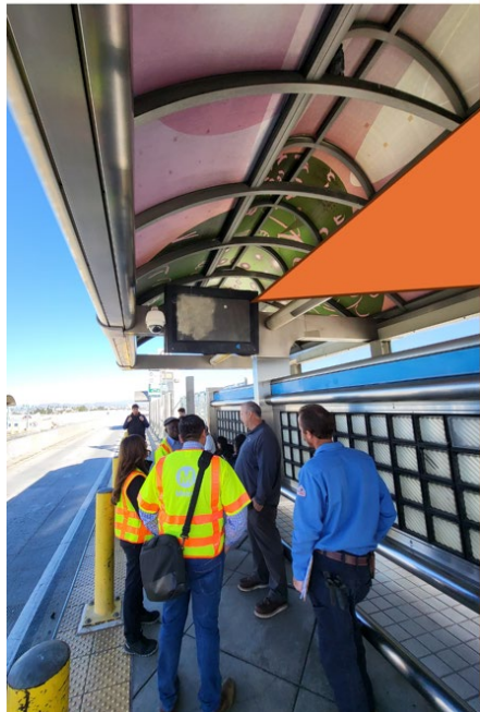
BEFORE: Persistent offenders would stand on the original bench partitions to steal real-time digital displays and cables, then re-wire extension cords to the hiding area behind for unauthorized use, resulting in loss of customer information and $10,000+ in damage.
