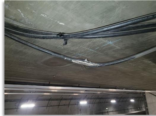
Failed feeder cable securement
