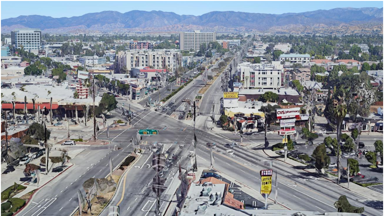
Figure ES-3 – North Hollywood – Vineland Avenue and Lankershim Boulevard Pre-Project
