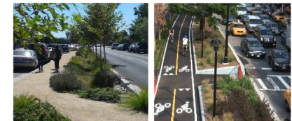
Examples of bioswale on pedestrian path (Woodman Ave) and between bikeway & thoroughfare (Queens Plaza Bikeway, NY)
