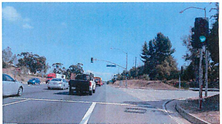
2 Southbound SR-71 & N. Ranch Road Intersection
