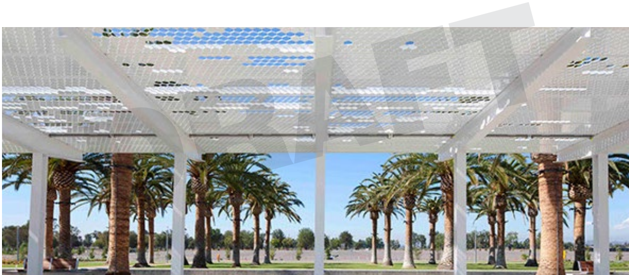
Perforated pattern in canopy creates interesting shade pattern on ground - Great Park, Irvine
