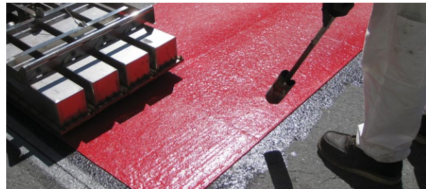
Thermoplastic Bus Lane Coating
