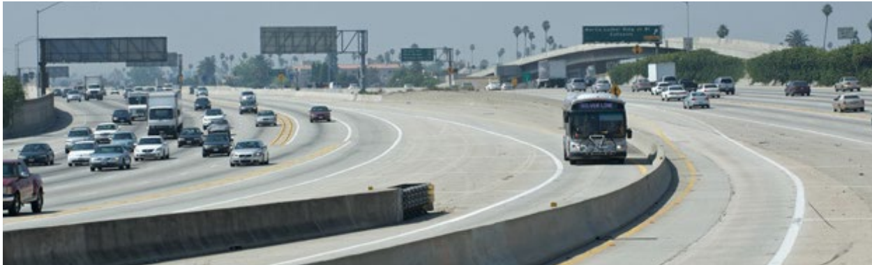
Figure 11. BRT managed lanes
