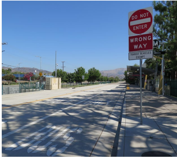
Figure 14. Exclusive BRT roadway
