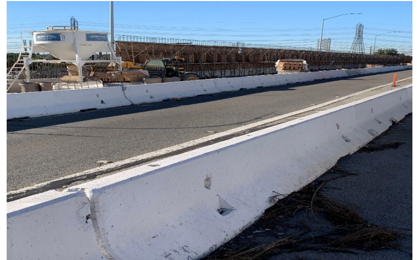
SB 405 Crenshaw Blvd off ramp (SW #815)
