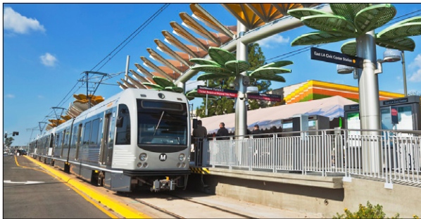
Figure ES-5: LRT High-Floor Example: Metro Gold Line
