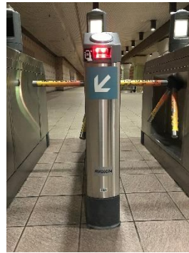
367 Gates 154 Emergency Gates
