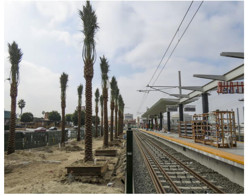
Downtown Inglewood Station – plaza, tracks and platform
