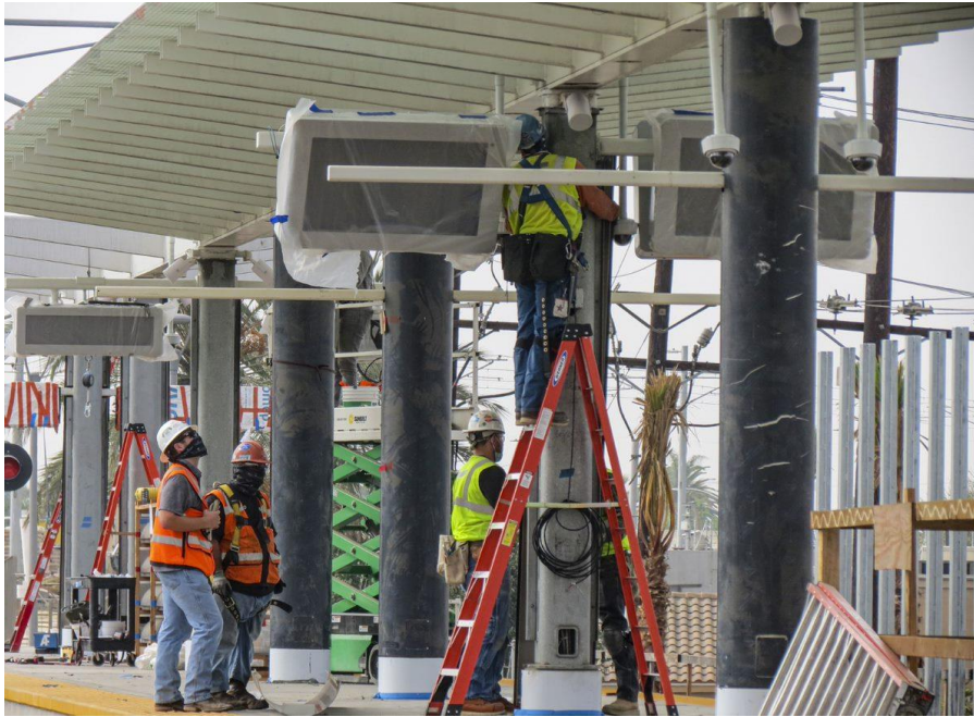
Downtown Inglewood Station – crews installing the platform LCD message screen
