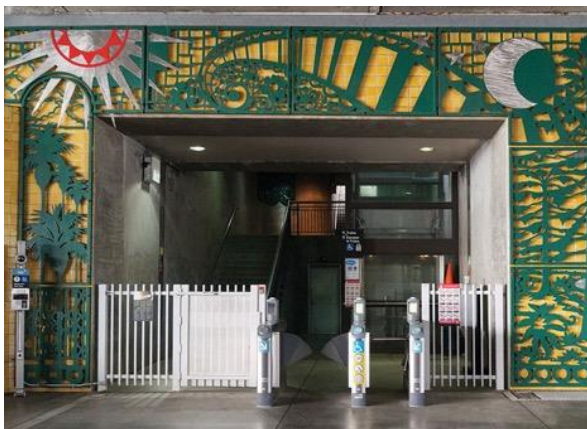
Allen Station Before
