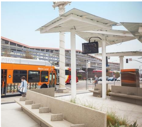
Routing and service frequency information on screens and in static signage at Chavez Pavilion, Los Angeles, Union Station.
