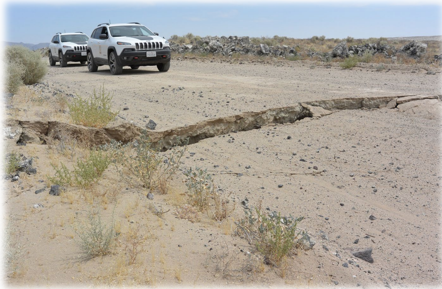
Caption: Fault rupture crosses dirt road, with California Geological Survey vehicles for scale. Displacement at this location is primarily normal (vertical). Photograph taken near the northern end of the rupture resulting from the M7.1 Searles Valley earthquake.
